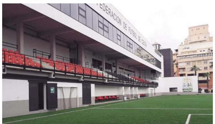
Headquarters of the Football Federation of Ceuta
