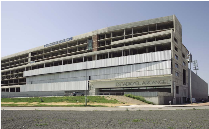
Offices Premises Stadium El Arcángel, Cordoba
