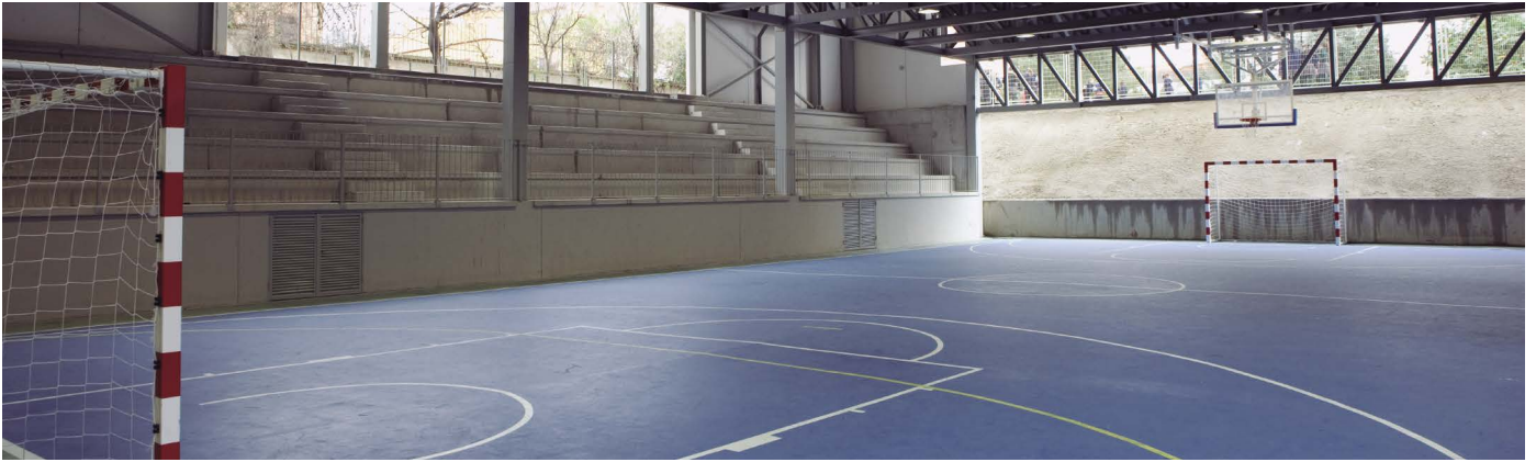
Roofed Tracks Nepomuceno School, Seville
