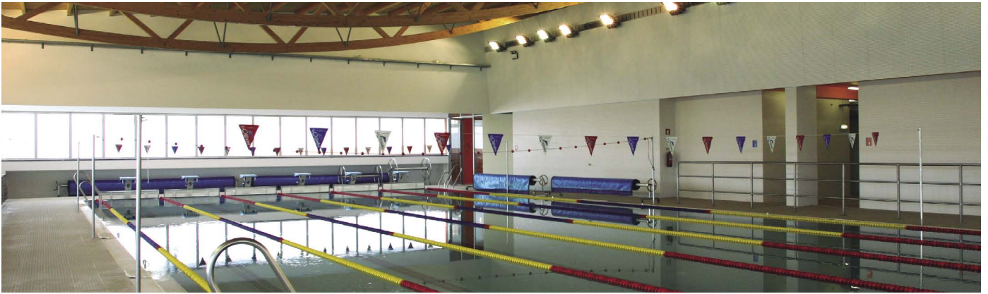
Municipal Swimming Pool of Sobreda (Portugal)
